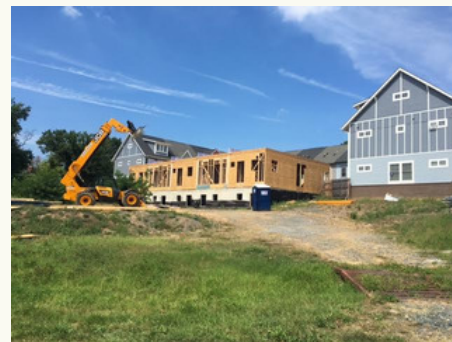
Eden Place Phase I Construction Sept. 2016
